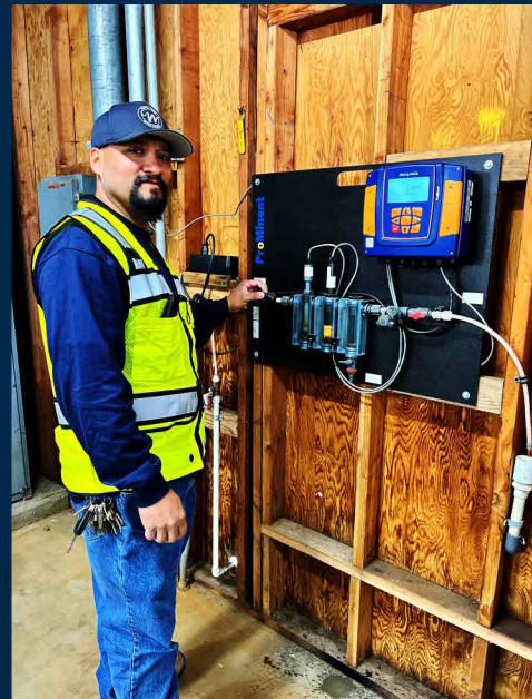
JOE PINEDA OPERATIONS & MAINTENANCE SUPERVISOR. 15 YEARS
